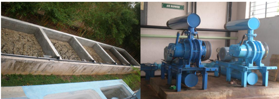
Fig. 7.5 Sludge bed and pump of sewage water treatment plant
